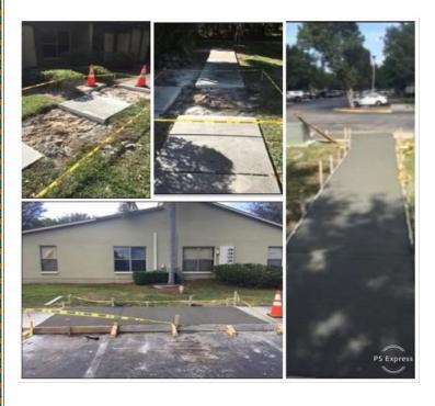
Work in Progress!! Concrete repairs to eliminate broken, cracked, and faulty sections. Rock and new soil added to eliminate eroded soil conditions.
